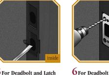
**5** For Deadbolt and Latch **Strikeplates:** Chisel out holes **Strikeplate:** Using reinforcing for dustboxes. Chisel out cavity strikeplate as a template, drill so deadbolt strikeplate and latch four 1/8" pilot holes for #8 x 3/4" strikeplate fit flush with doorframe. For deadbolt strikeplate, cavity is  $\frac{7}{32}$ " deep For latch strikeplate, cavity is
