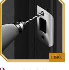
9 For Latch Strikeplate: Using latch strikeplate as a template, drill two 1/8" pilot holes
