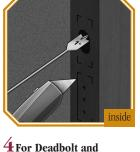
Latch Strikeplates: Mark drill points 5/16" above and below center points. Bore two 1" holes 1¼" deep for deadbolt dustbox and two 1" holes 1" deep for latch dustbox. Score chisel guide into door frame with utility knife.
