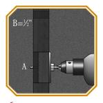
Complete drilling hole (A) from opposite side of door. Drill (B) ½" hole into door exactly at pencil mark.
