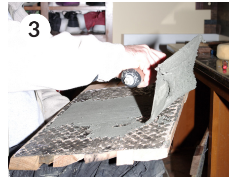
3 Use a 3/16" V-Notch Trowel and spread the adhesive evenly over the back of each wood piece as well as on the surface in which it will be mounted.
